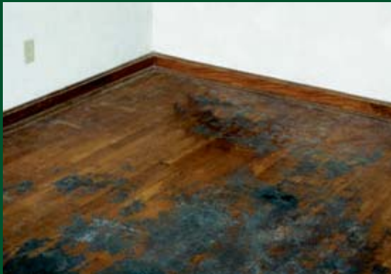
Water or pet stains (pet stains may not come out even after total resanding).
