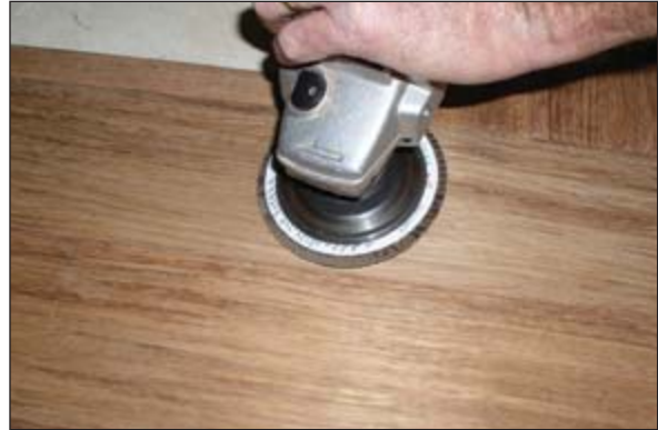
A 4-inch circular grinder creates dish out.
