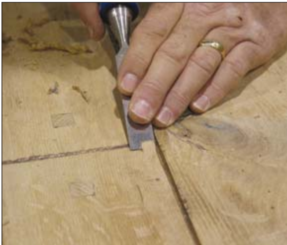
Using a chisel to create chips.
